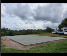
SHED SLAB BROOM FINISH
