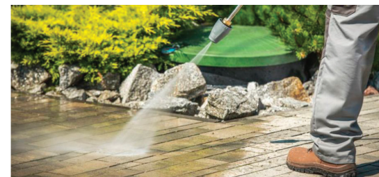
High Pressure Water Blasting
